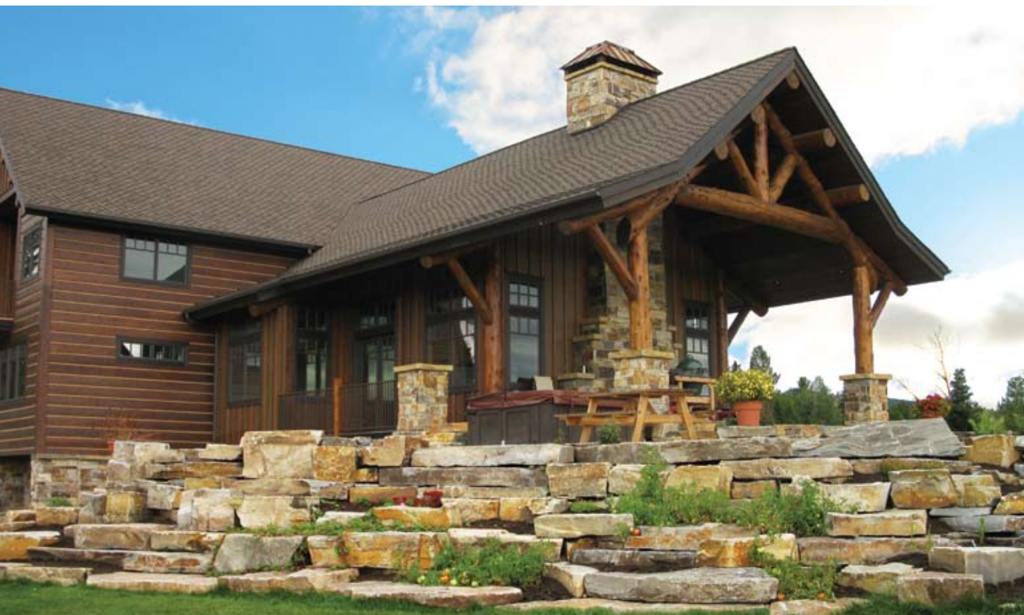
52 | Montana Rockworks, Inc — 2015
